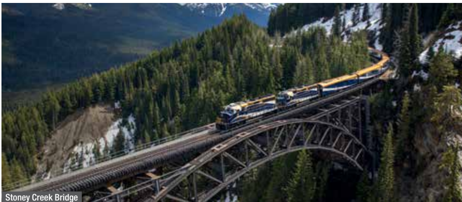
Stoney Creek Bridge
