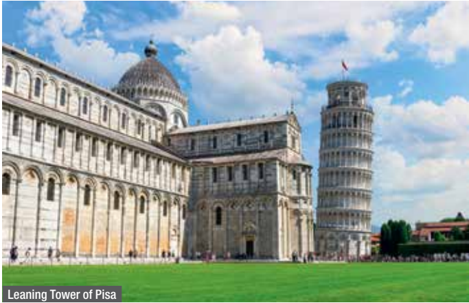
Leaning Tower of Pisa
