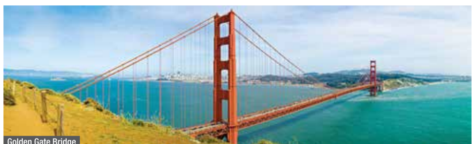
Golden Gate Bridge
