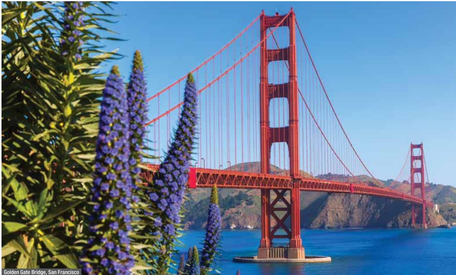
Golden Gate Bridge, San Francisco
